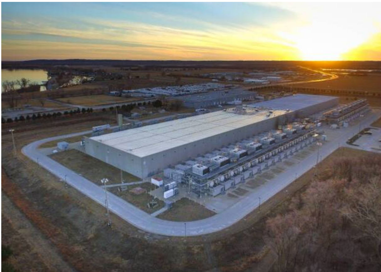
Google Data Center, Council Bluffs Iowa
