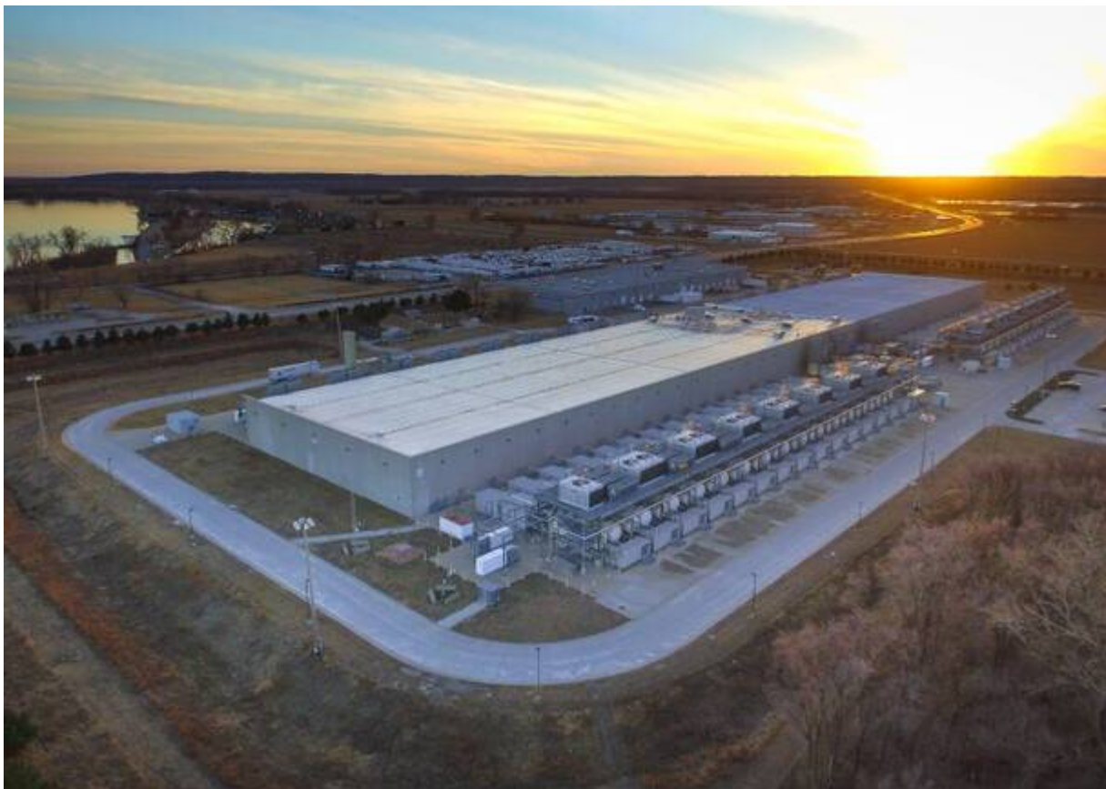
Google Data Center, Council Bluffs Iowa, foto wikimedia
